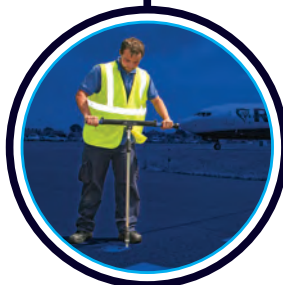
MALMS Engineer Records replaced lights
